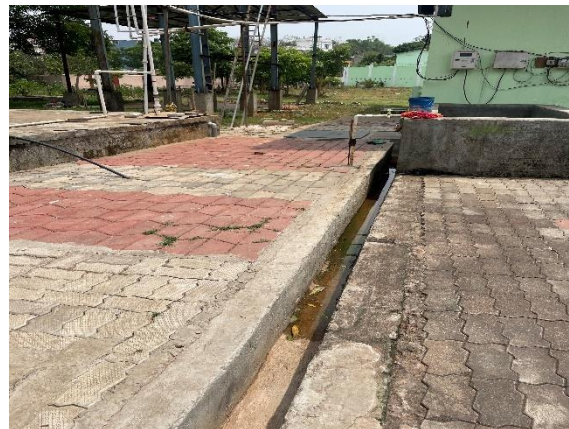
Washing area for cleaning the utensils and kitchen tools. The area has proper drainage with inlet and outlet water delivery.
