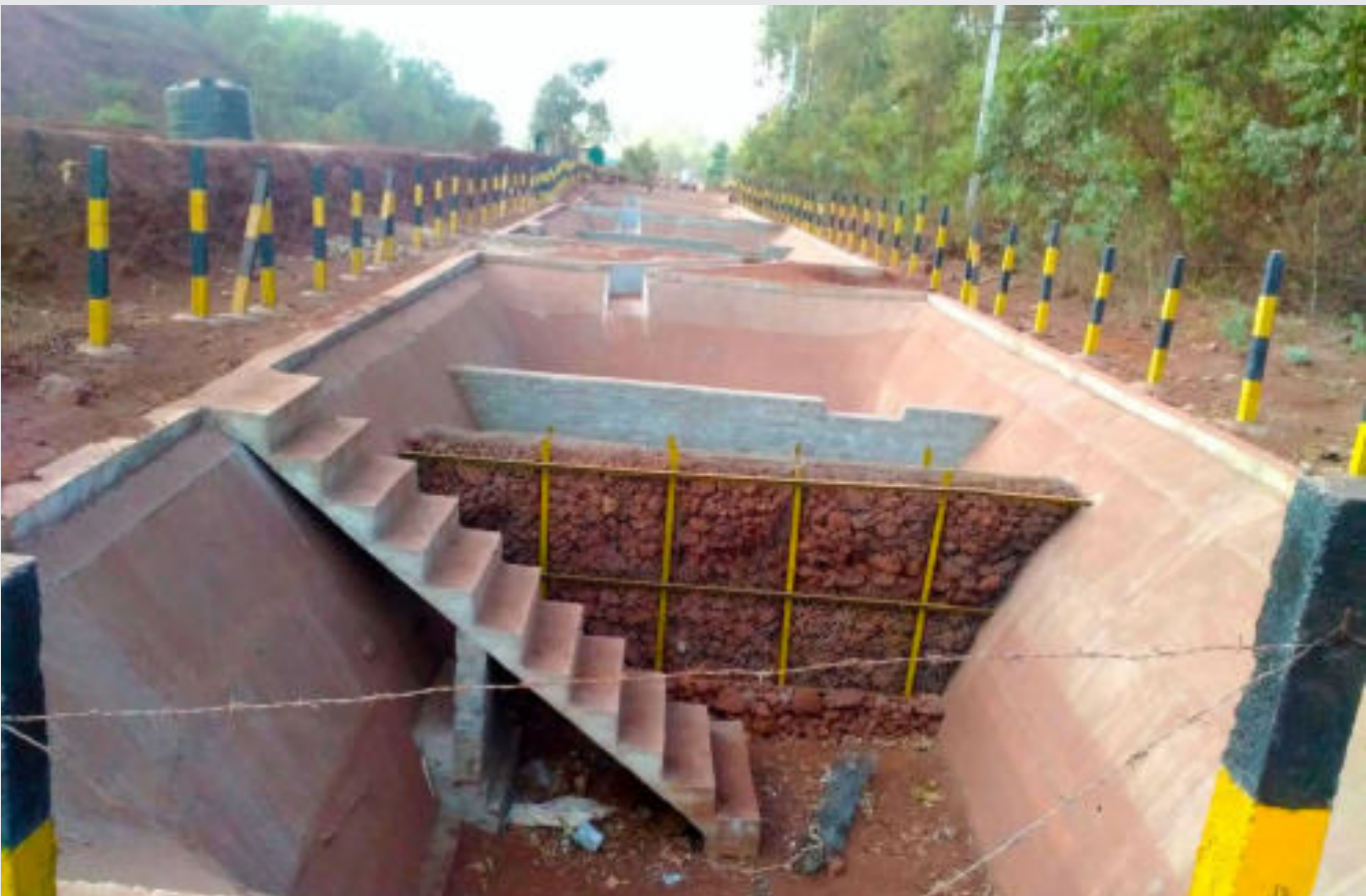
Storage cum percolation tanks at Koira Mine
